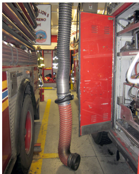
This hose draws out carbon monoxide fumes that build up from idling engines inside the fire station. In prior times, carbon monoxide fumes and diesel exhaust caused cancer and other serious illness in some firefighters.
